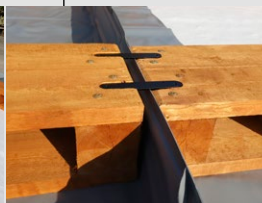
Detail of anchorage of a wooden ramp
